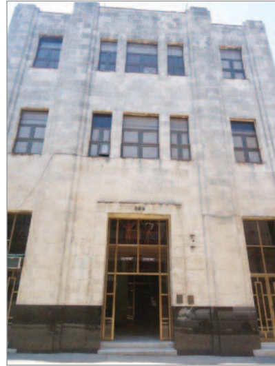
INIMET building in Cuba
