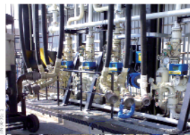
Calibration of a road tanker loading rack in a fuel storage plant
